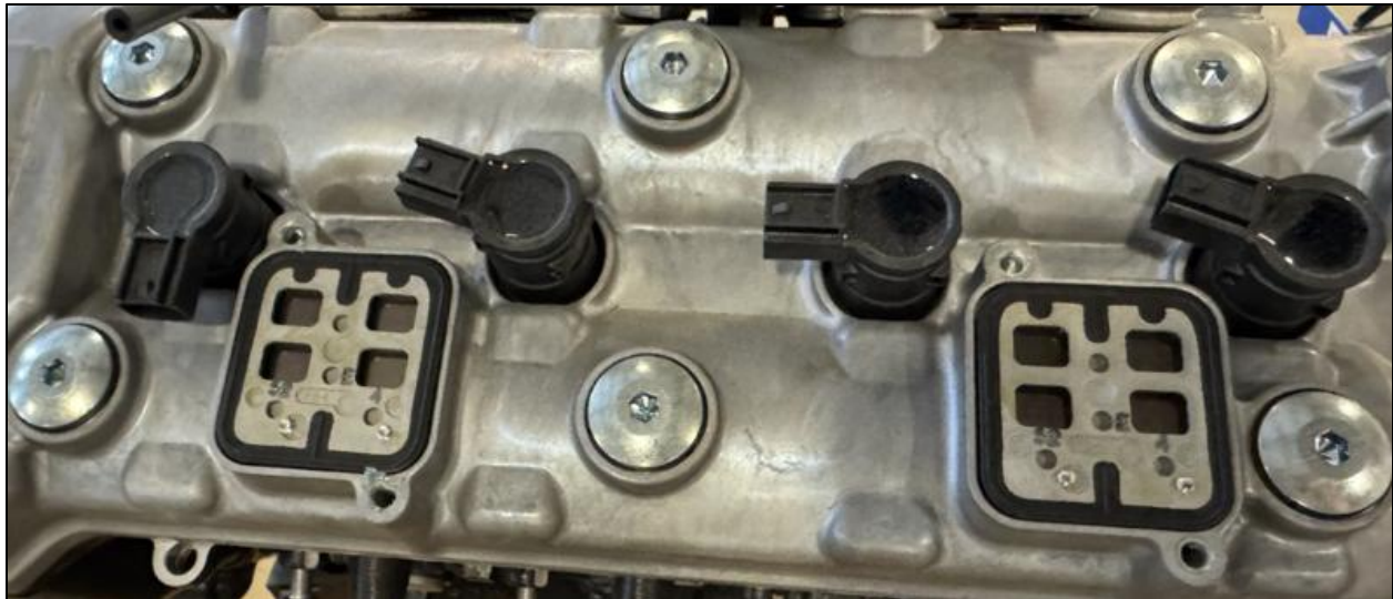
Figure 21: Recirculation Caps Removed
