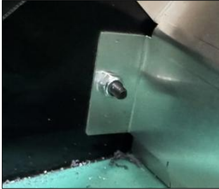
Figure 19: Bottom Bulkhead Connection to Side Panels
